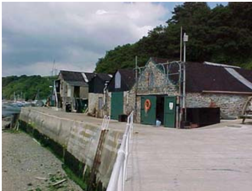
Brazen Island maintenance yard
