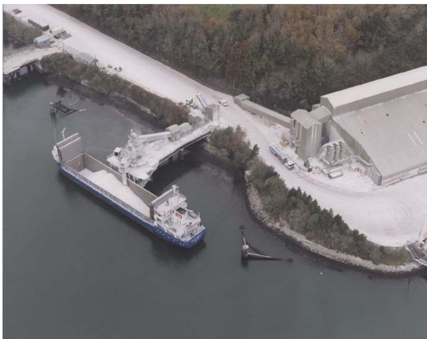
Aerial view of a wharf operated by IMERYYS Minerals Limited
