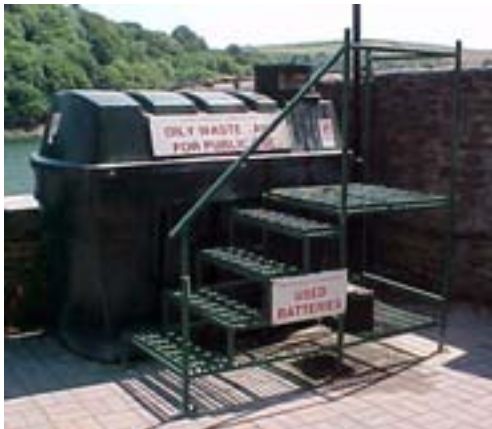
Oily Waste Receptacle at Berrills Yard
