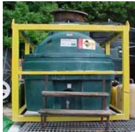
Self bunded tank at Brazen Island
